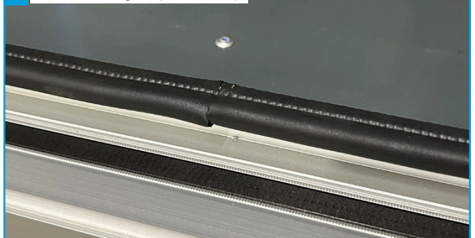
7 End of Sealing Strip Butted-up
