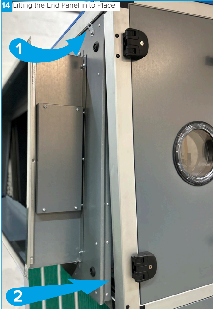
15 End Panel Lifting Lugs
