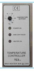
POWER - YELLOW AIRFLOW FAILED - RED HEATER ON - RED
